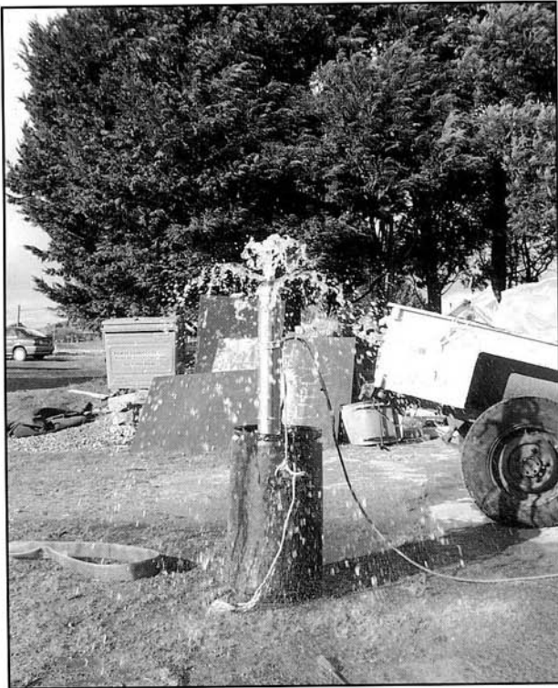
The bore hole pump being tested.
