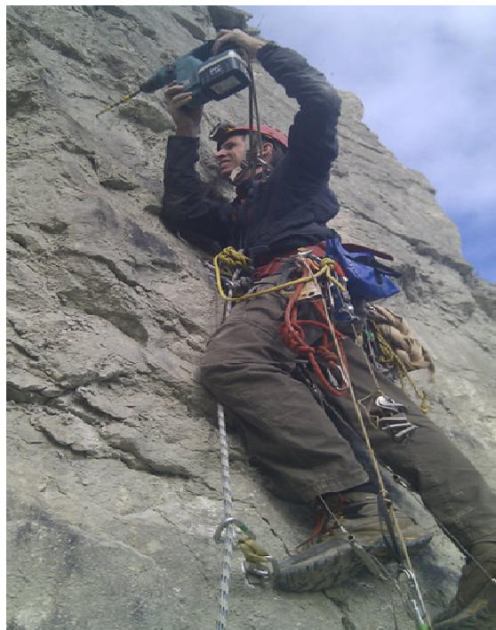
Alan practicing bolt placement
